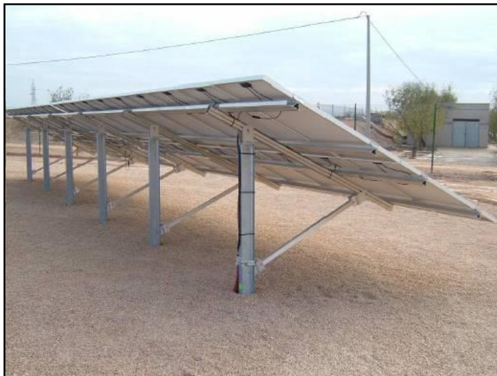
Figure 3-5: Rear View of a Typical Ground Mount Support Structure
