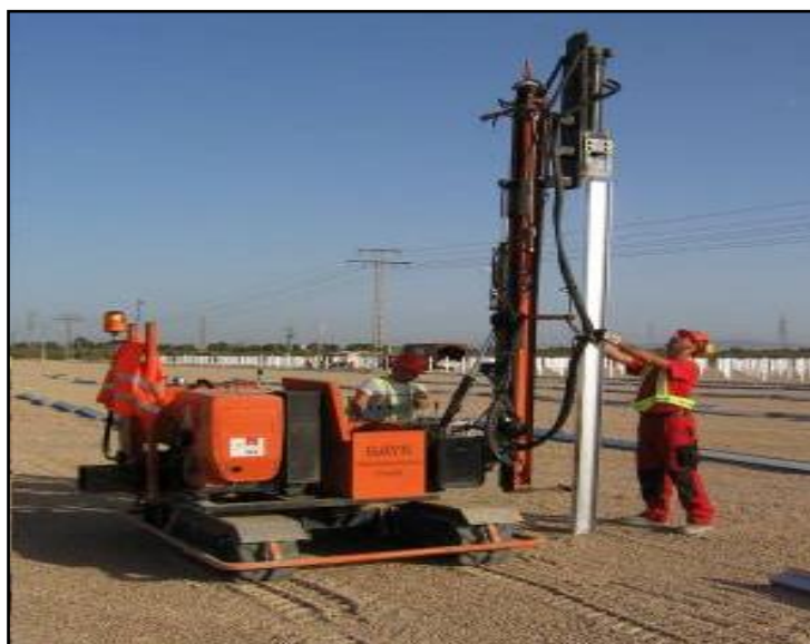
Figure 3-6: Hydraulic Driving Machine for Installing Piles
