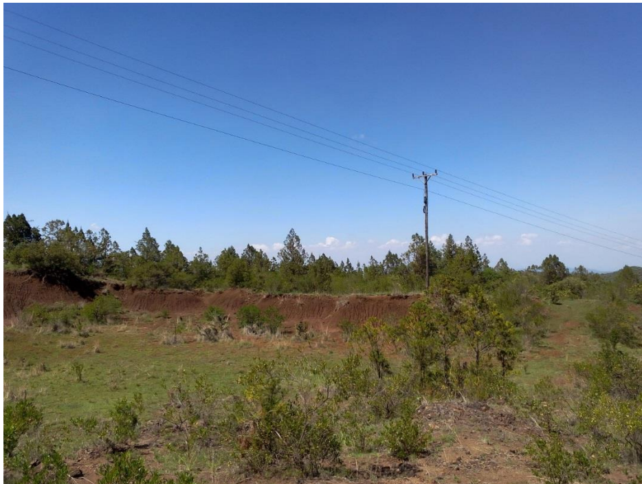
Figure 6-16 - Nanyuki-isiolo-Meru 33 kV power line
